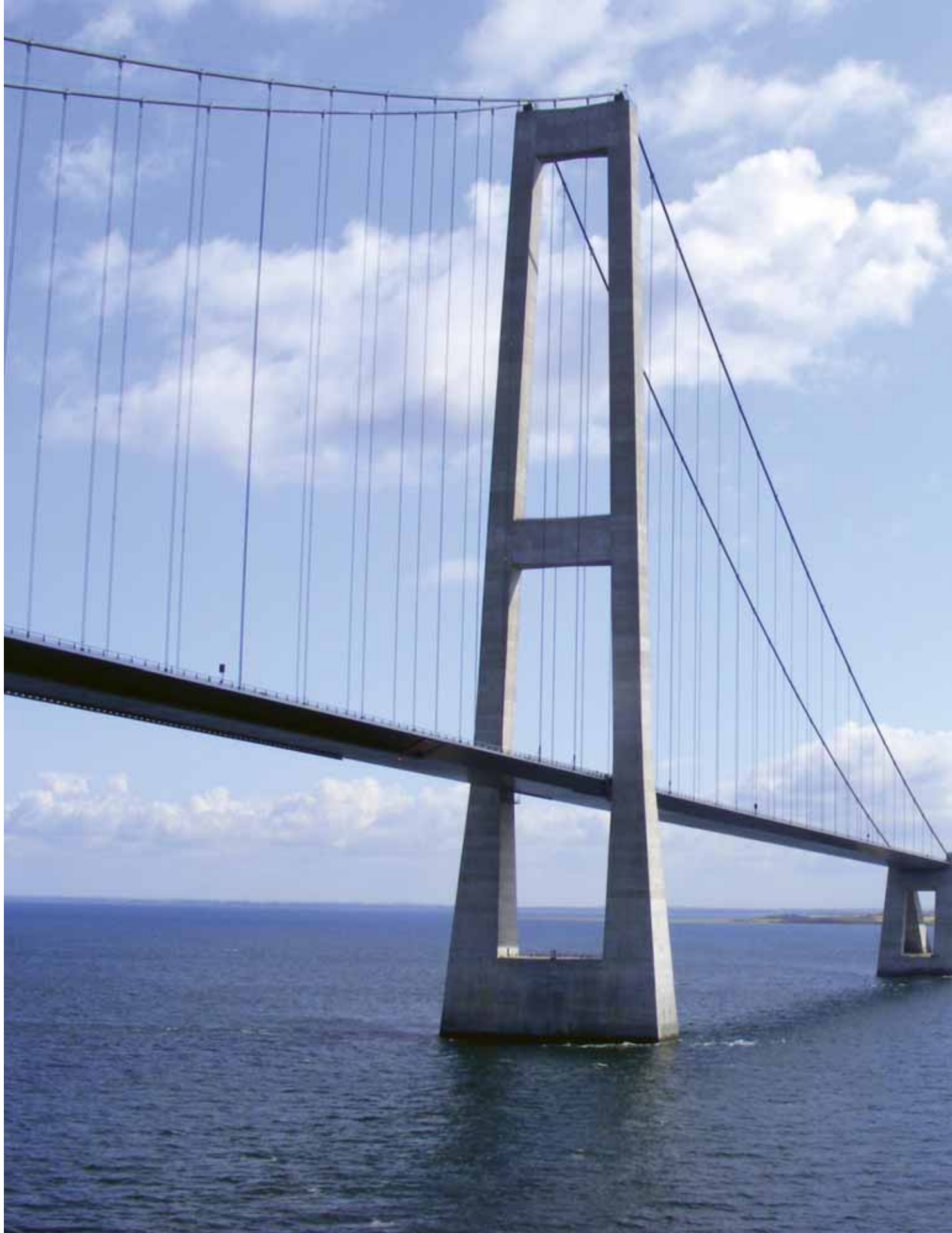
The Great Belt Bridge ZEALAND – FUNEN, DENMARK – 1998 http://www.storebaelt.dk/english/about
