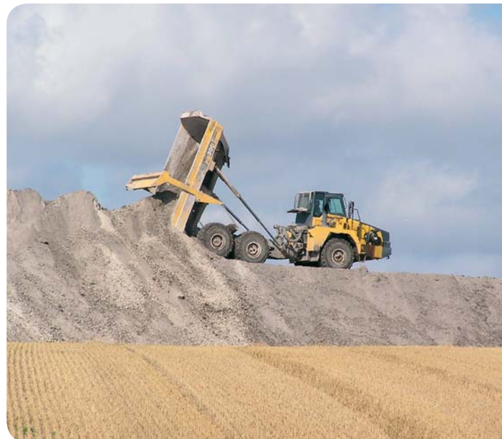
Extension of noise embankment at Øster Uttrup
