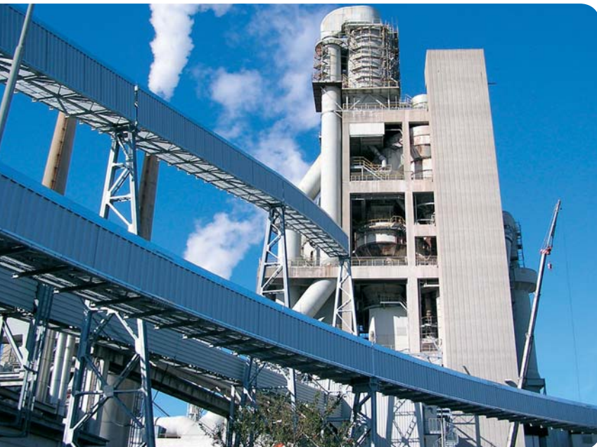
Noise suppression of feed to Kiln 87 by enclosure of conveyor installation
